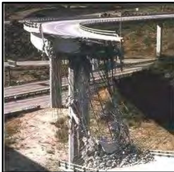
Surface waves caused this freeway off ramp to break apart and collapse in during an early morning earthquake in California.
